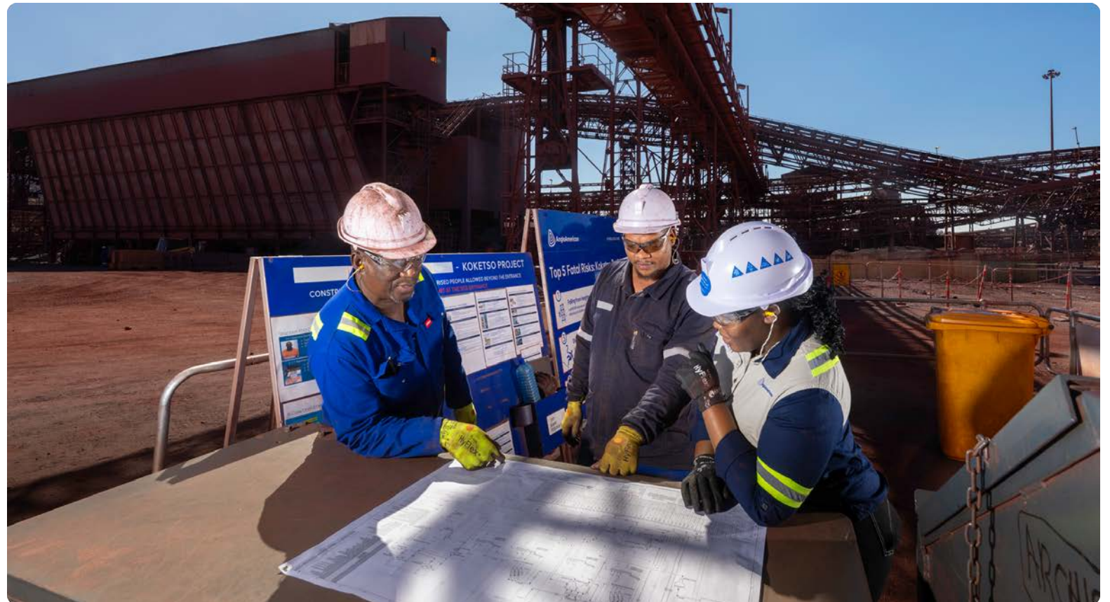
The UHDMS project will convert the current DMS processing plant at Sishen to UHDMS technology. This technology uses specialised ferrosilicon in the plant processing of raw iron ore and allows greater flexibility to process a wider range of Fe grades and densities. The implementation of the technology will improve the proportion of premium iron ore and lower the waste stripping ratio, while maintaining the Lump:Fine ratio. Seen here are Tsheulo Reginald Ntau, Supervisor Drum Processing, Pretty Molele Mailula, Radio Communication Officer, and Neo Renigious Osile, Operator Grade 1.
