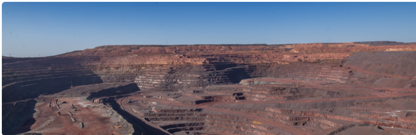
Sishen mine, North Pit - also referred to as G80. Pushback 5 (left side of the picture) is active as it transitions from pre-strip waste mining to internal waste and ore exposure. In-pit dumping is visible to the right of the mined-out pushbacks. This reduces the mining footprint and reduces diesel consumption and carbon emissions.
