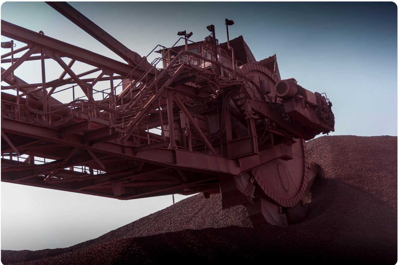
Reclaimer in operation on lump ore product stockpile at Kolomela mine.
