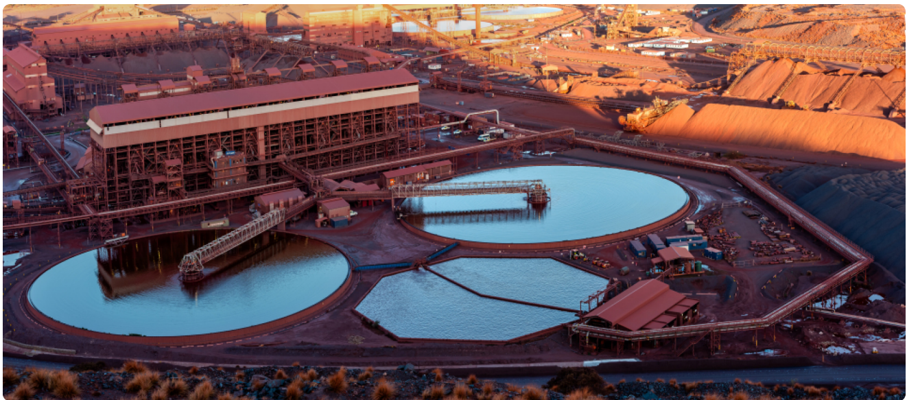
Sishen mine DMS and Jig beneficiation plants, with the settling dams.
