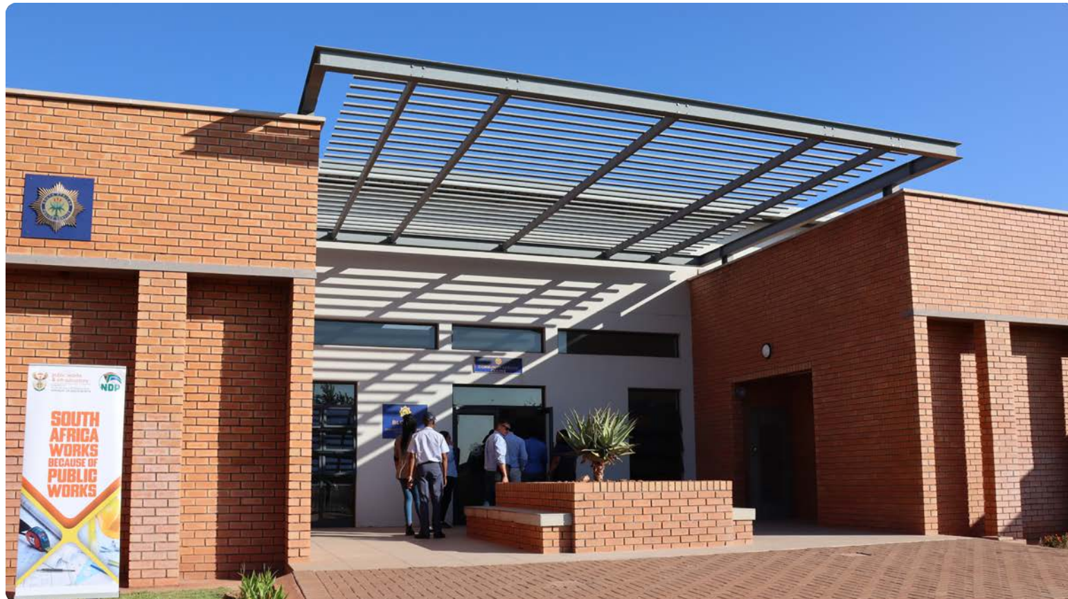
Handover of the Siyathemba Police Station to the community.
