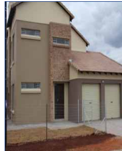
Pensfontein housing development
