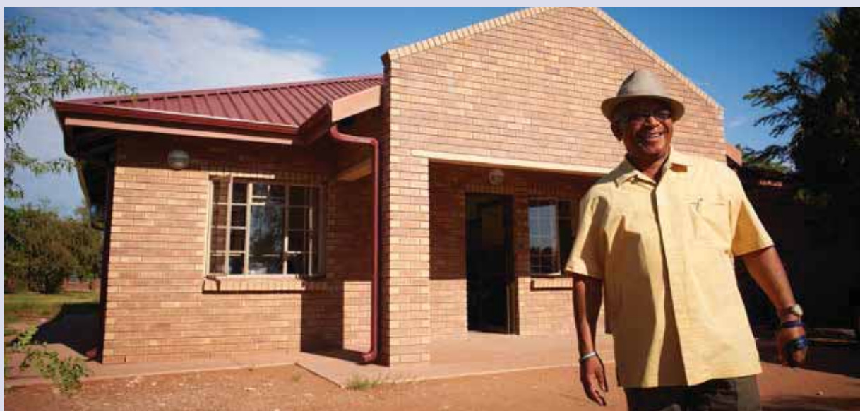
Mr Okhau in front of one of the newly constructed buildings at the Sishen Intermediate School in Sesheng.
