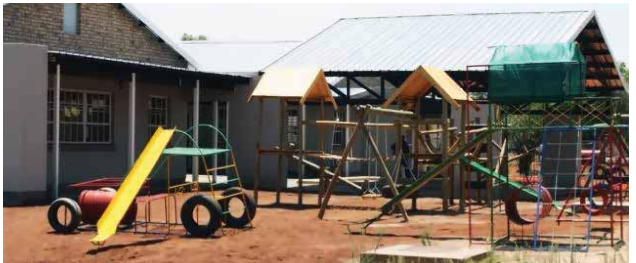
The new Grade R facilities at the Asmandia Primary School.
