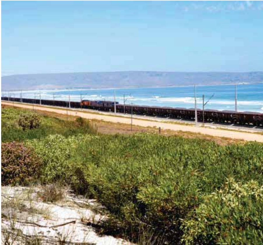
The 861km rail system that links the Sishen mine to Saldanha port is among the most efficient and advanced logistical systems in the world.
