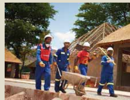
Patrick Moletsane, Dumisani Ndlovu, Abram Maletswa and Petros Tuis, four builders working at the Thabazimbi Cultural Village construction site.
