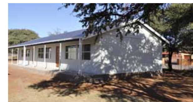
New classrooms have been built to cater for the growing learner numbers of Kathu High School.
