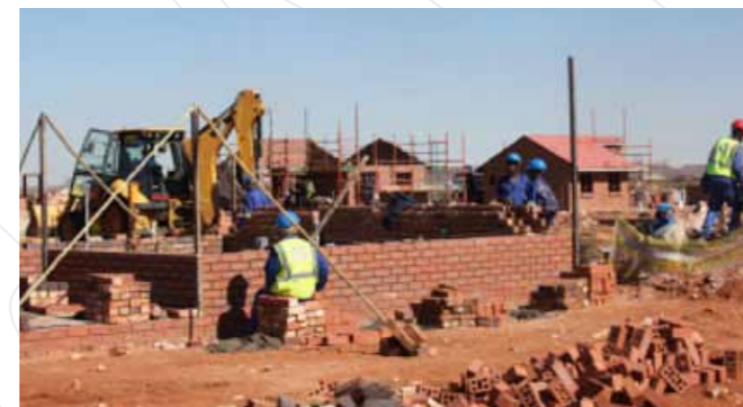
The foundation walls for the first of 49 municipal houses.
