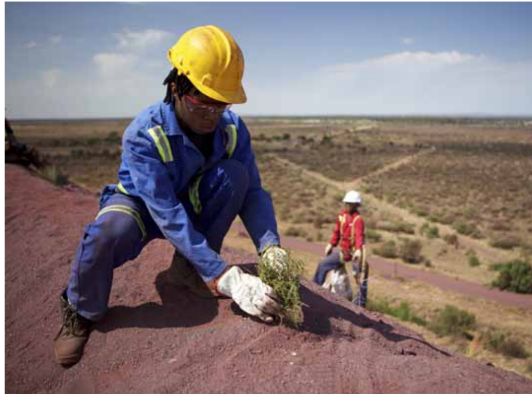
Lesego Mase (foreground) and Alfred Douf on the slope of the waste rock dump at area G60 in Sishen. Grass is planted on the slopes to bind the soil.
