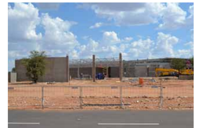
The new Checkers mall is currently under construction in Kathu.
