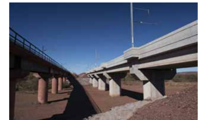
As part of the South Western Expansion project at Sishen, a railway line has had to be moved to allow for the widening of the pit. The rail line footprint has had to be widened and bridges have had to be constructed to allow for this.
