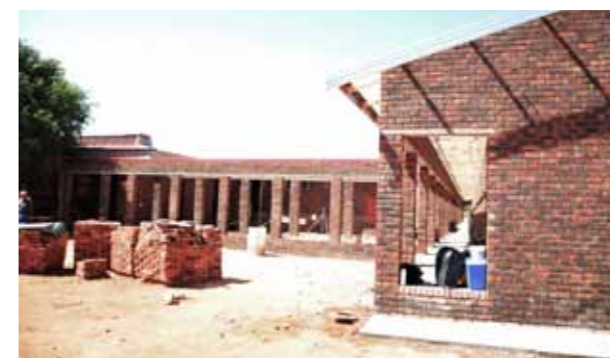
Construction work at Sesheng Intermediate.
