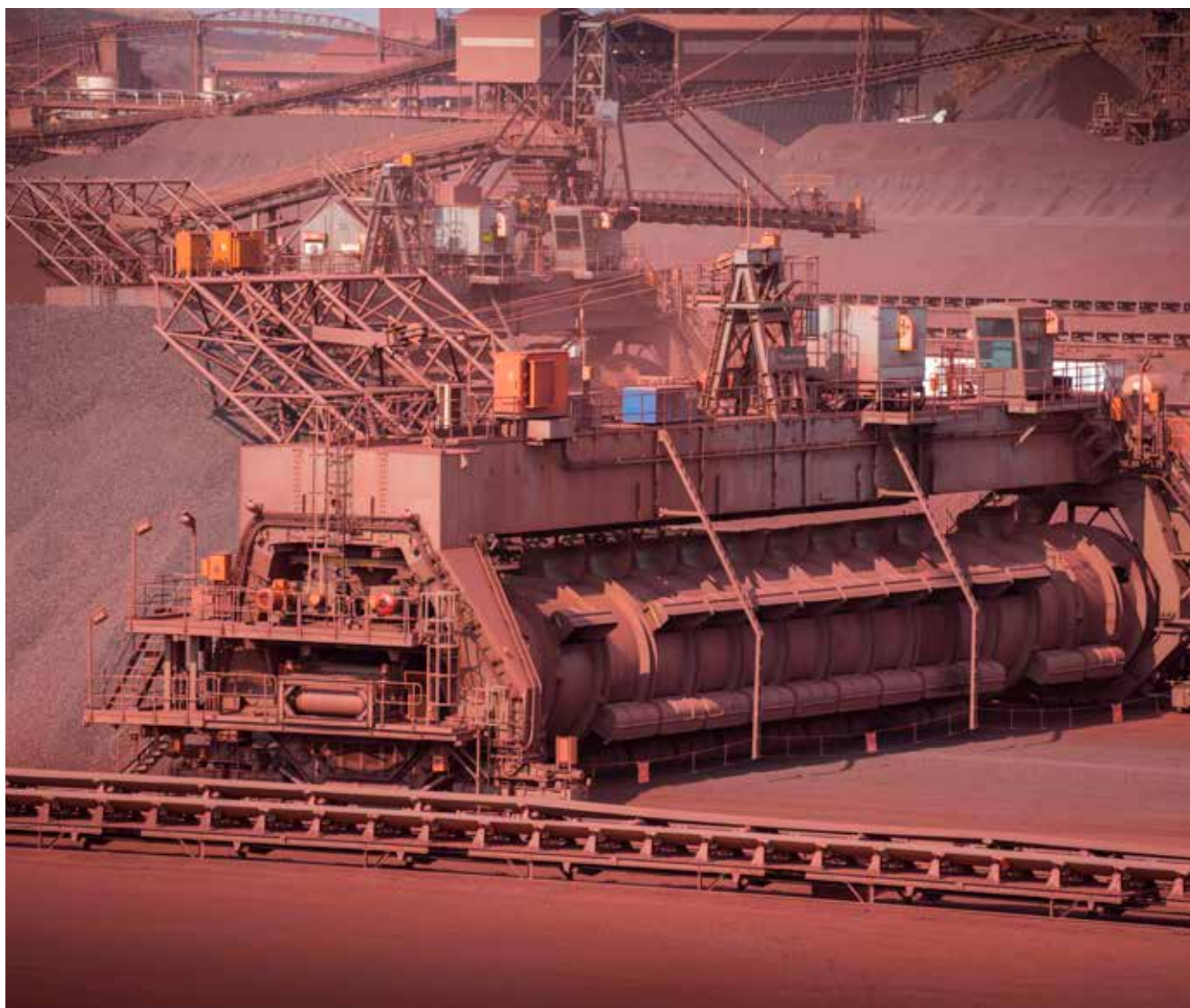
Image: General view of the DMS plant at Kolomela mine.
