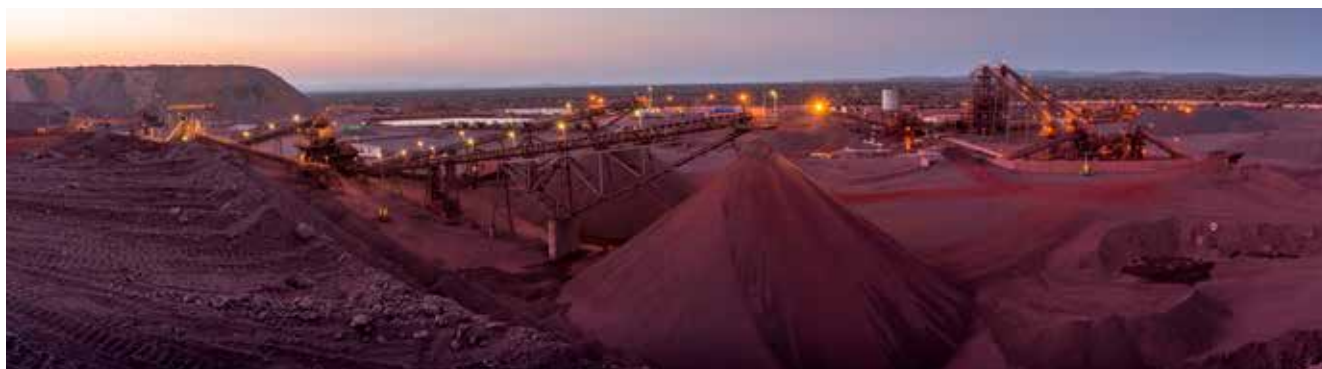
Image: General view of the plant and load out station at Sishen mine.
