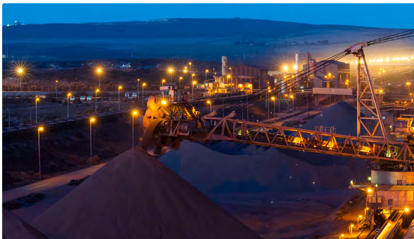
General view of the stacker reclaimer in the ore stockyard.
